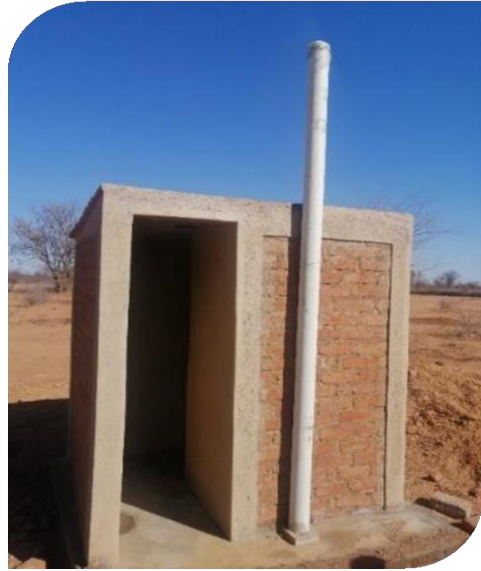
Blair ventilated improved pit (BVIP) in Nkayi
